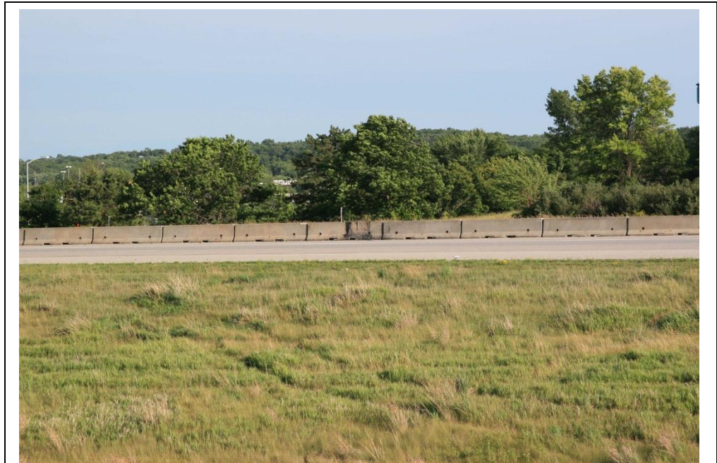
Exhibit 2. Concrete median of F-shape barriers at site
