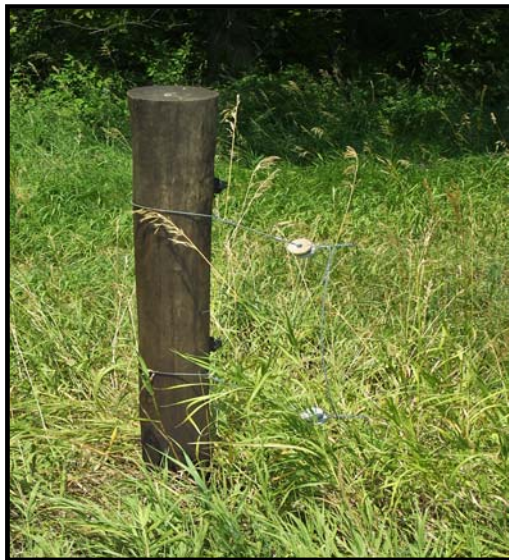
Photo 4 – Wooden fence post, similar to the one in the incident.
