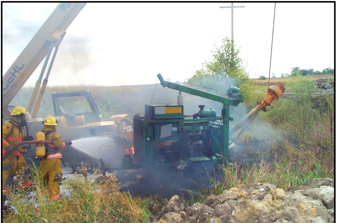
Photo 2 – Second view of firefighters at the scene, showing the portable hydraulic power unit and the suspended
