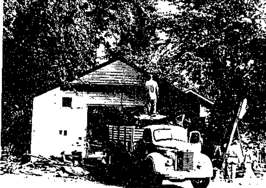
Figure B13. Tearing down Little Ankeny in 1953, south view. The building was used shortly after World War II for the production of thorium and for other particularly dirty processes. By 1953, it had outlived its usefulness and as Harley A. Wilhelm succinctly put it, "it had become more reactive than active."
